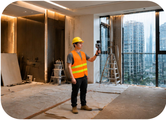
Interior Design and Refurbishment
